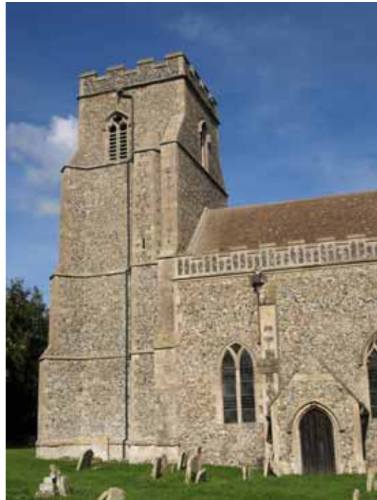
St Peter's Church Tower
