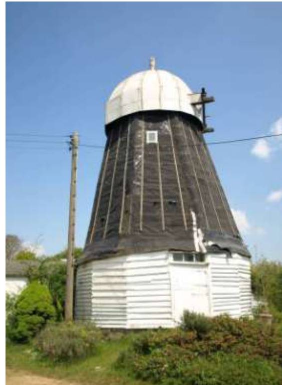
Overhead Wiring and Mill
