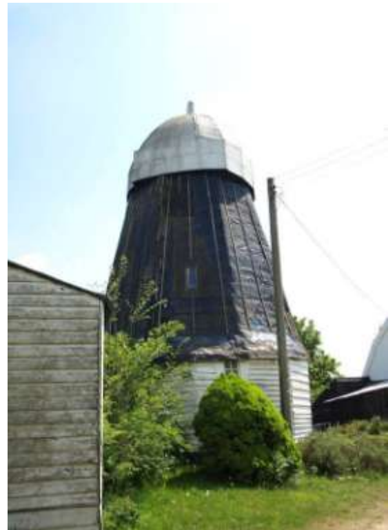
Temporarily Clad Smock Mill
