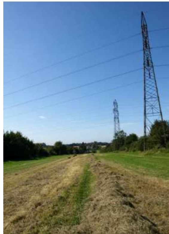
Pylons over Badley Walk
