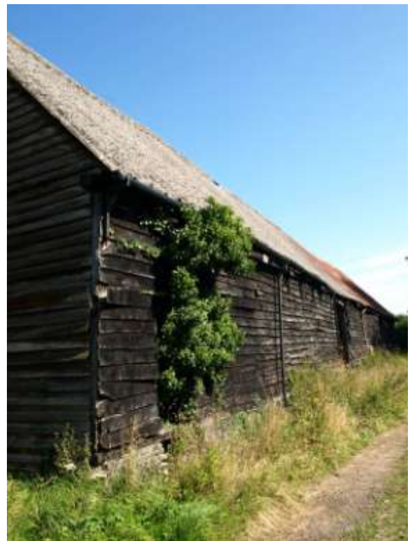
Asbestos Roofing
